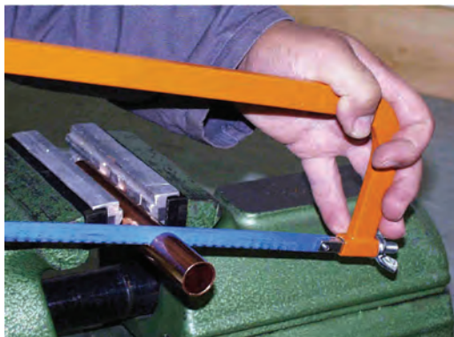
1. Rectangularly saw off the pipes
